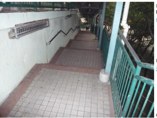
Handrail not covering the entire length of staircase
