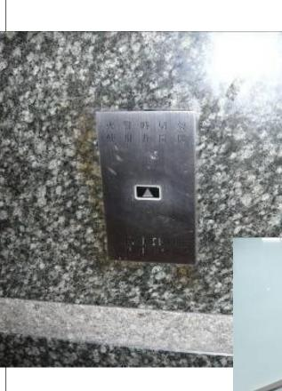
No Braille and tactile control buttons installed
