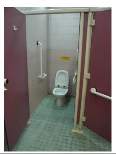
Insufficient space inside 'accessible toilet' (1040mm(W) X 1500 mm(L))
