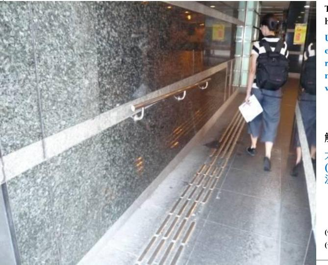
Tactile guide path too close to handrail
