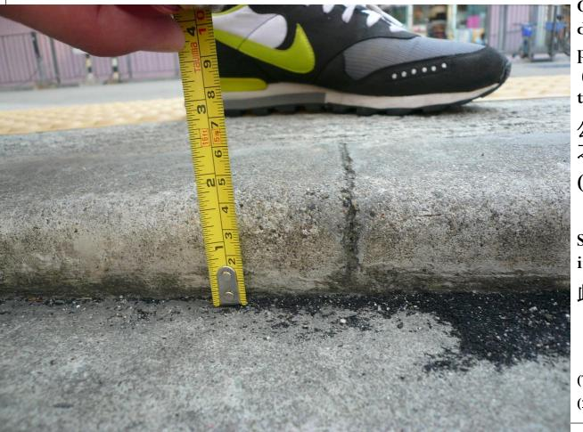
Great level difference (35mm) at dropped kerb connecting pavement and road service (DM 2008: difference not greater than 15mm)
