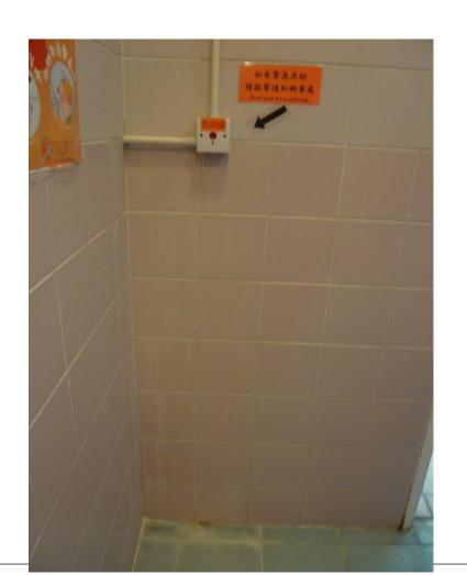
Emergency call bell installed outside accessible cubicle and at 1420mm high
