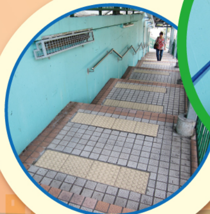
Example of Barriers: Non-provision of handrail at some sections of the staircase
