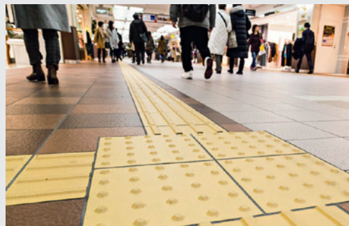
上圖：為視障人士鋪設的引導徑 Photo above: Tactile guide path for persons with visual impairment
